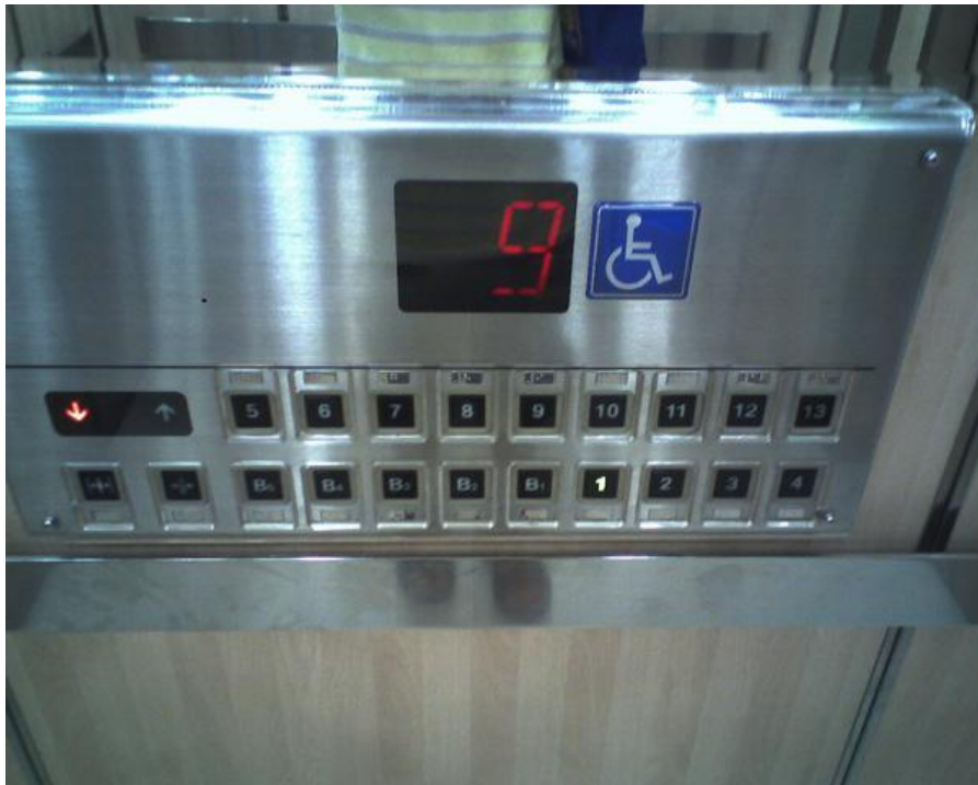
Figure 9: A Handicapped Panel in Elevator
